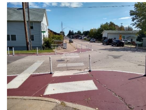
Demonstration project in Proctor – The project slows traffic and shortens the distance between curbs, which improves visibility and makes it safer and more comfortable for people walking.
