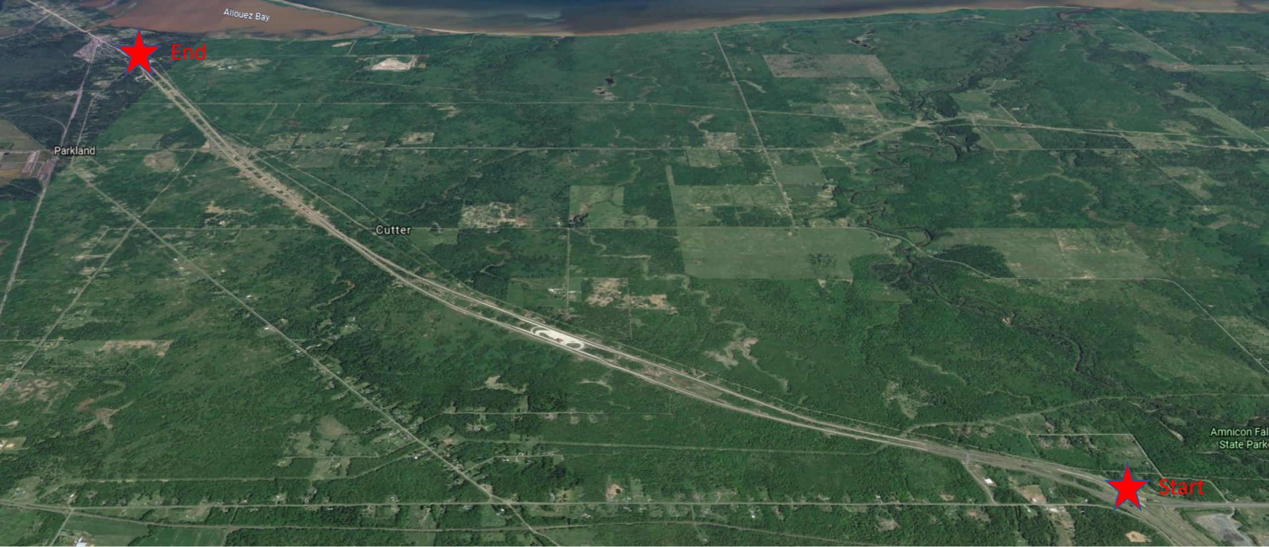
113-19-014 – USH 2/53: Interchange to Moccasin Mike Rd. 2019 – Repairs due to buckling - Const. - $64,000
