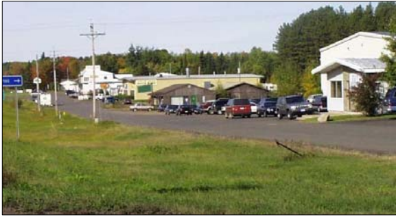
Figure 1d: Service road connecting to Lavaque Road.
