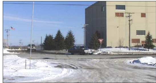
Figure 2b: The Airport Road intersection is unsafe due to its limited sight distance and a small median crossover.
