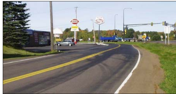
Figure 1a: Service road near the Midway Road/TH 53 intersection.
